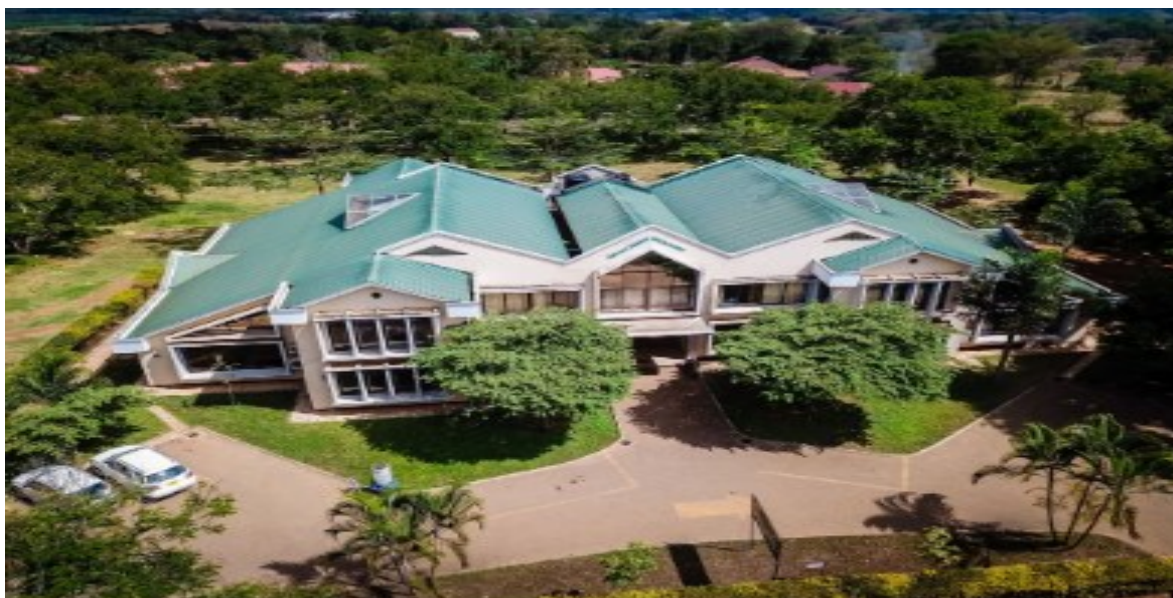
Figure 23: The aerial view of the National Carbon Monitoring Centre at SUA
