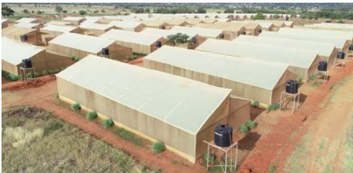
Figure 24: Some of the greenhouses built under the SUA-PASS collaboration
